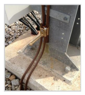
DSA Copperweld<sup>®</sup> wire and strand have the high currentcarrying capacity characteristics in short-time durations, high strength properties and corrosion resistance to effectively and economically meet IEEE recommendations. These advantages are particularly evident when compared to a low-strength material such as solid copper. Solid copper conductors must be upsized in many installations to meet the mechanical demands within a system design.
